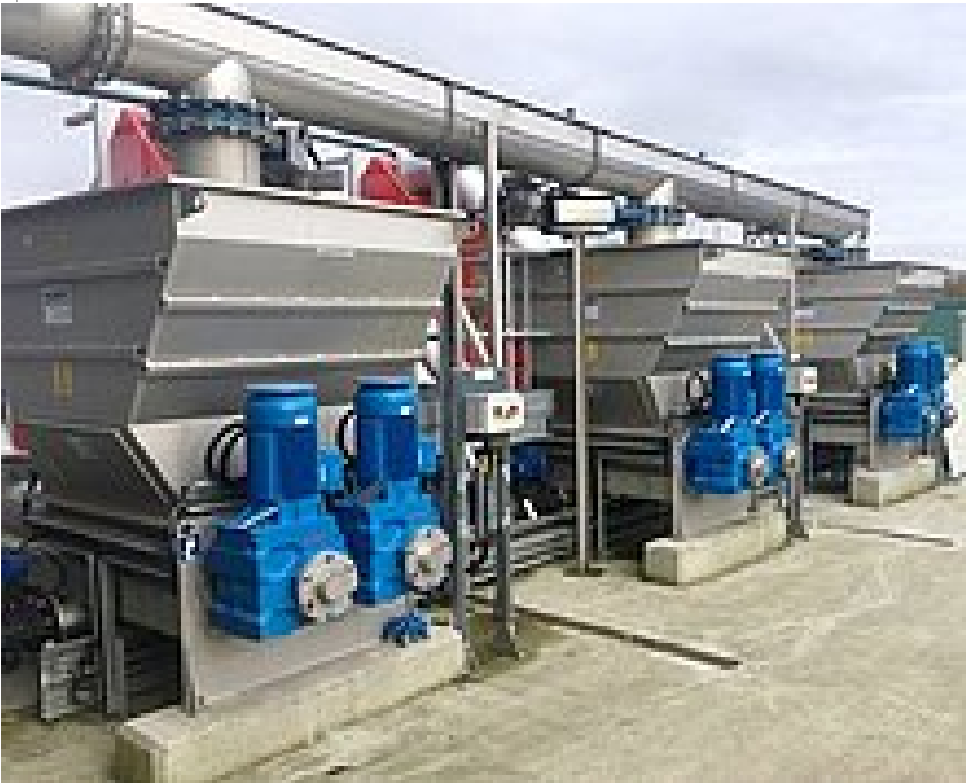
Fine screens low level launder and WAP® SL 12v wash presses
