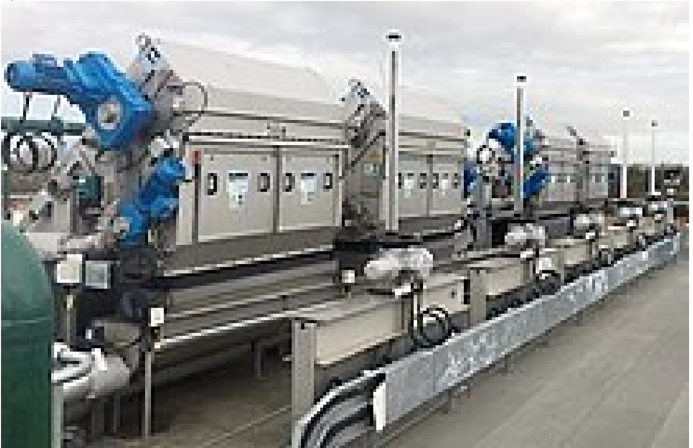
HUBER Belt Screen EscaMax®, 6 mm perforated plate screens
