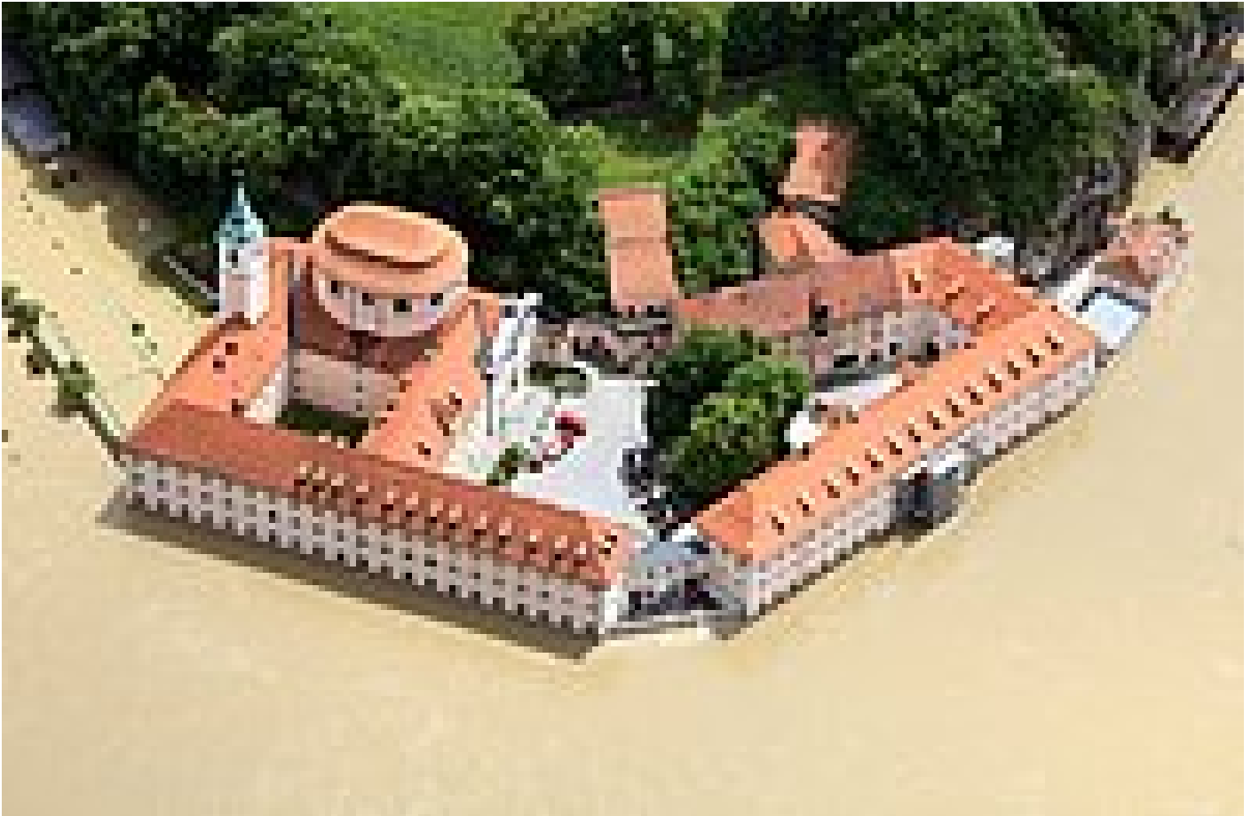
Weltenburg Abbey during the heavy storm flood in June 2013 (image rights: Weltenburg Abbey)
